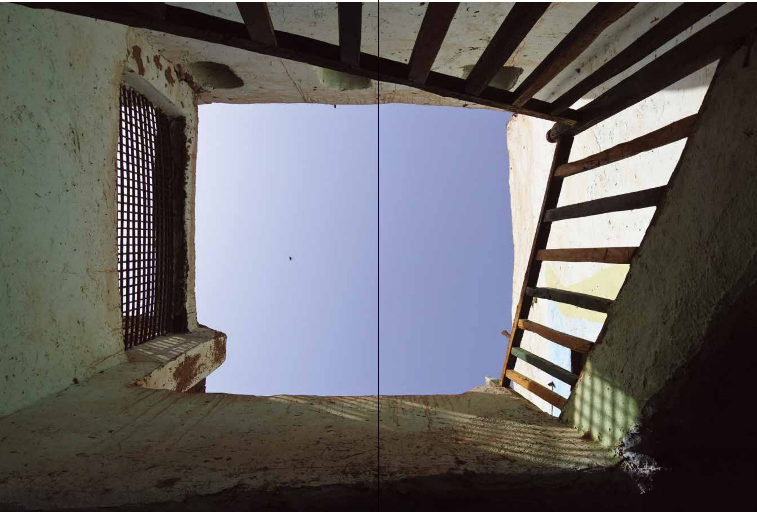
The atrium of a rural house in Gezira, Luxor West Bank. Photo: Zs. Vasáros, 2019.
