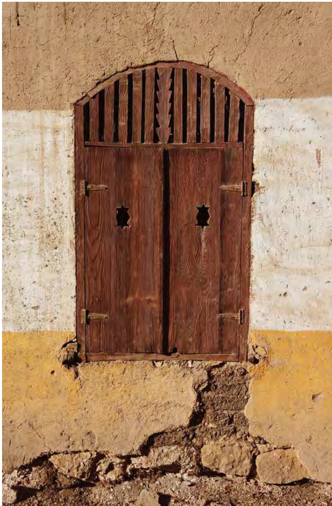
A window of the Village Hall. Photo: Zs. Vasáros, 2017.
