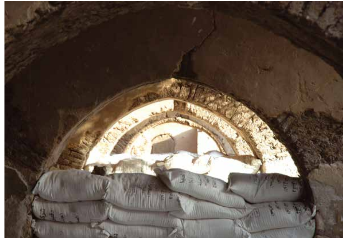
Temporary use of the former stables. Photo: Zs. Vasáros, 2015.
