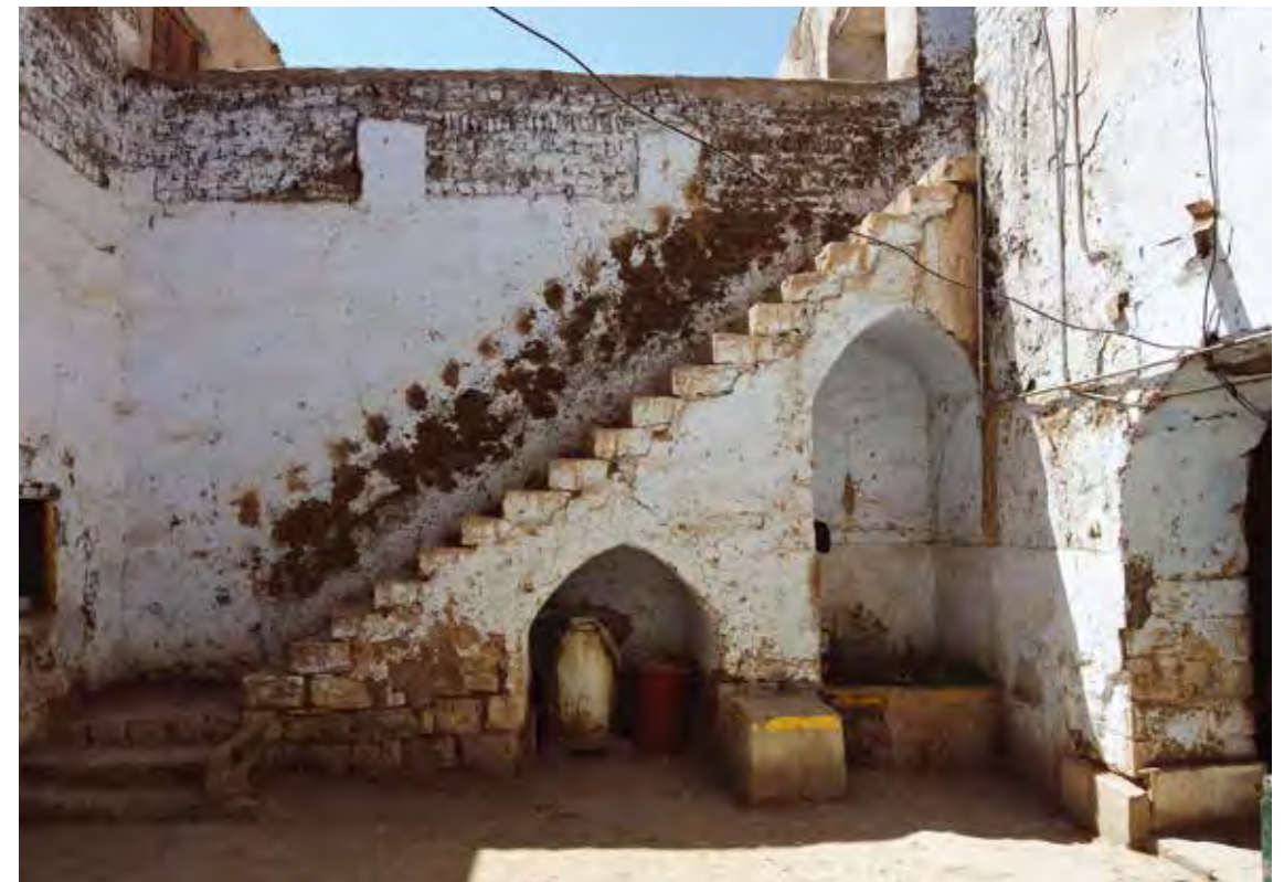
The second courtyard of the former Omda's House these days. Photo: Zs. Vasáros, 2017.
