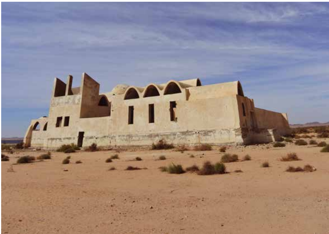
The Sadat Rest House. Photo: Zs. Vasáros, 2017.
