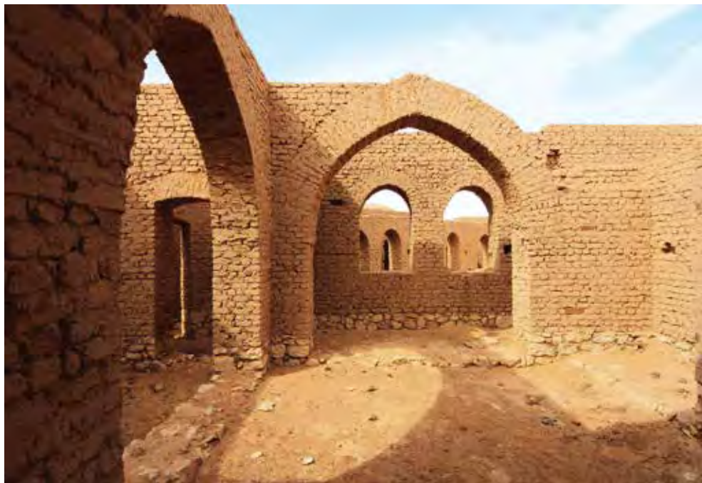
Unfinished building in New Baris. Photo: Zs. Vasáros, 2015.
