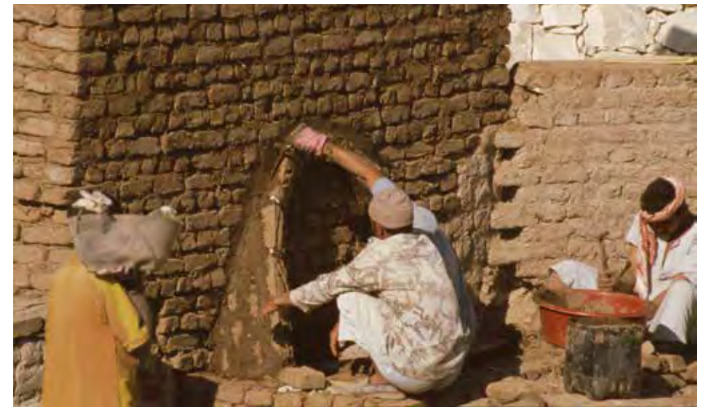
Reconstruction works of the Late Period tomb on El-Khokha in the Necropolis of the Noblemen in Luxor West Bank. The tomb was excavated by the Hungarian Archaeological Mission in Thebes under the supervision of Prof. L. Kákósy and Dr. G. Schreiber. Parts of the unique structure were built with Nubian vaults. 76 Photo: Zs. Vasáros, 2004.
