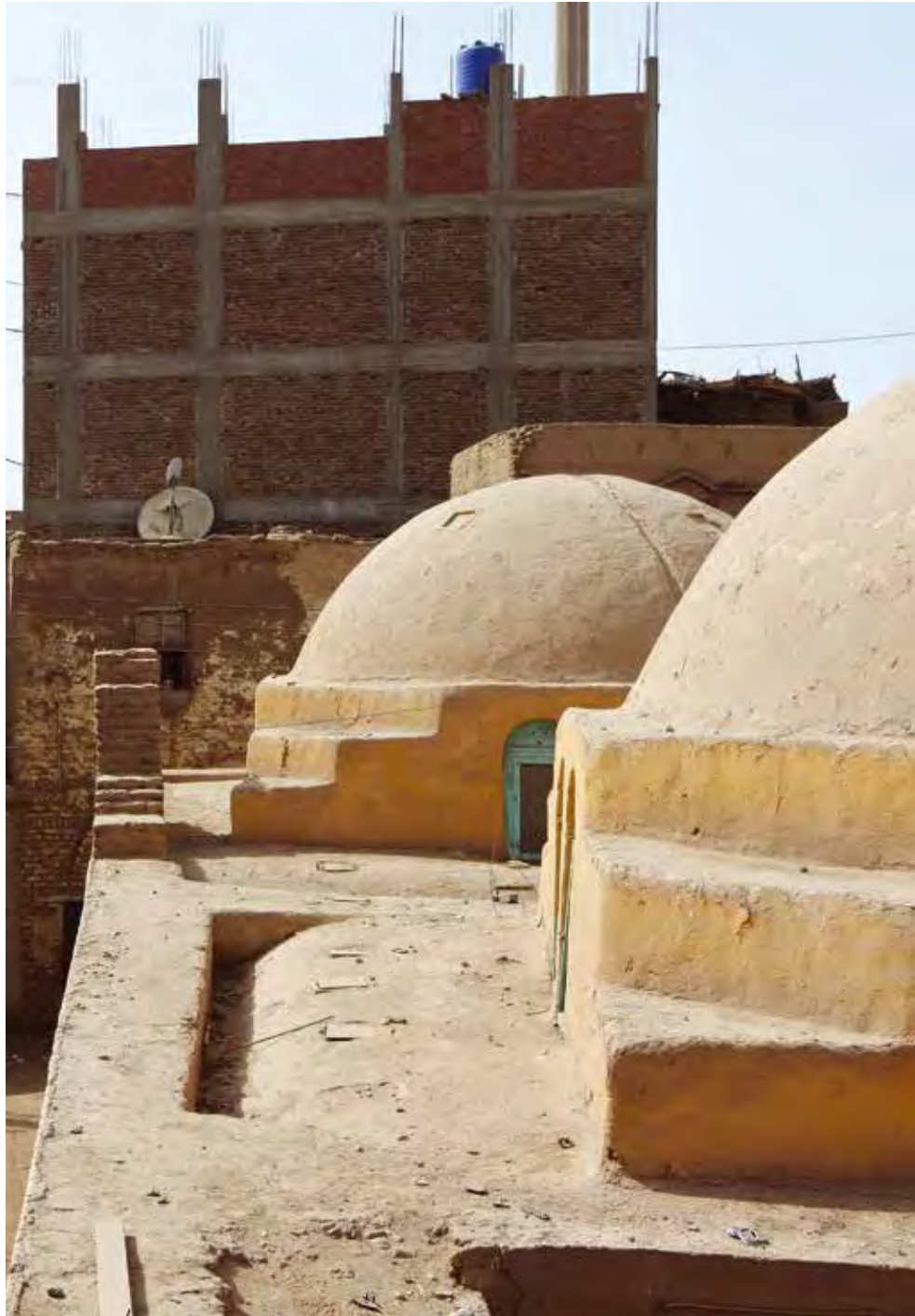
Rooftop of the school. Photo: Zs. Vasáros, 2017.
