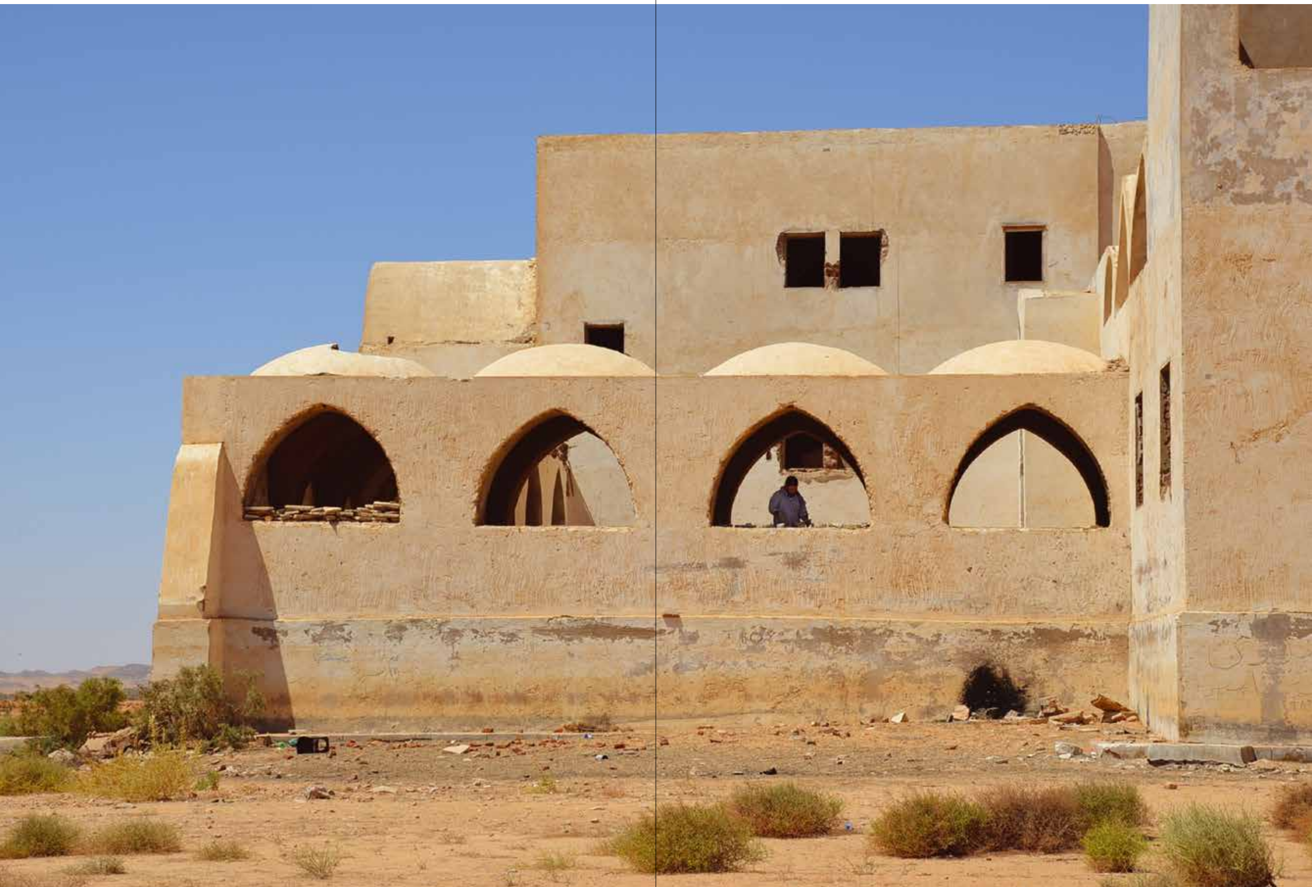
Façade detail of the Sadat Rest House. Photo: L. Veres, 2017.
