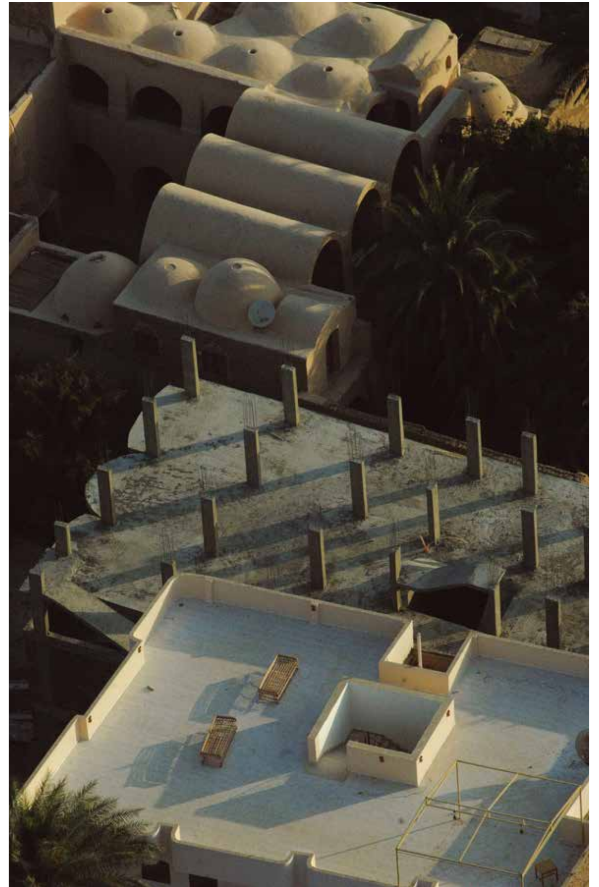
Domed-vaulted structures and the typical reinforced concrete and burnt brick architecture in Luxor West Bank. Photo: Zs. Vasáros, 2011.
