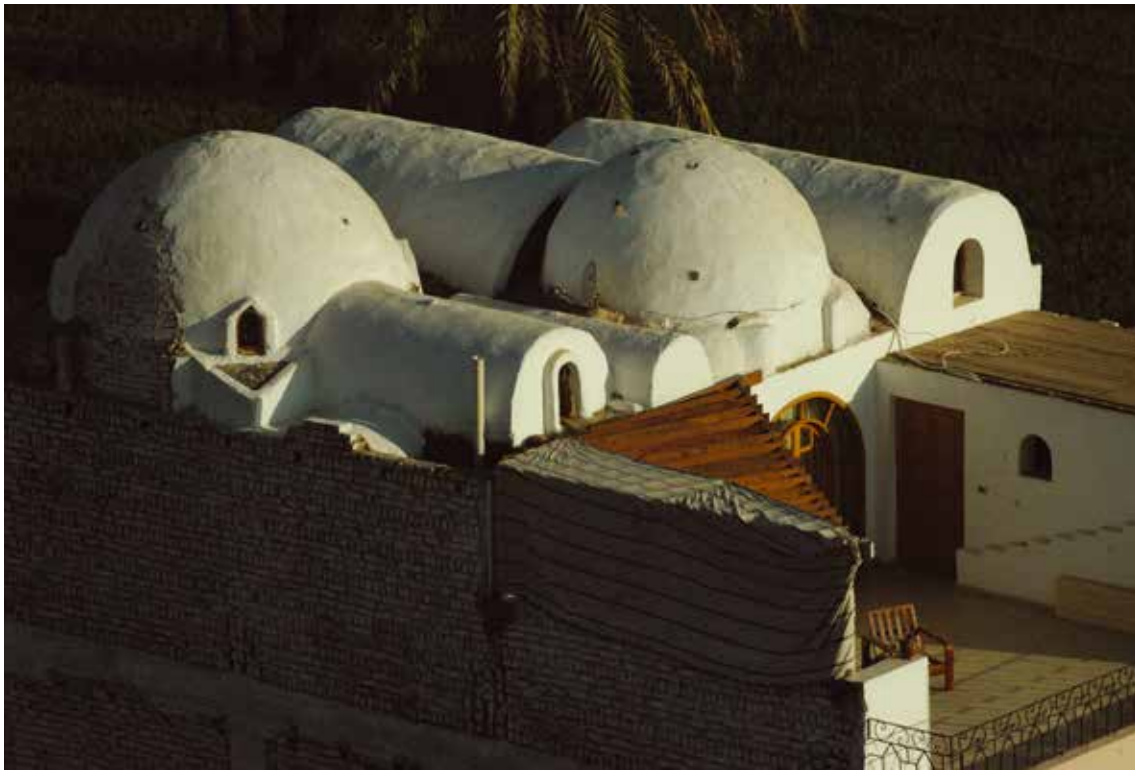
Domed-vaulted architecture in Luxor West Bank. Photo: Zs. Vasáros, 2011.
