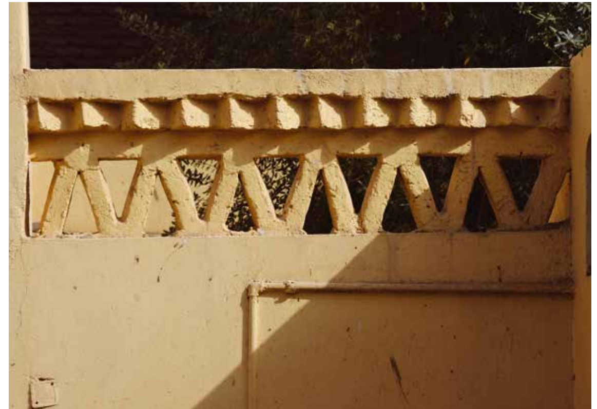
Façade ornaments. Photo: Zs. Vasáros, 2017.
