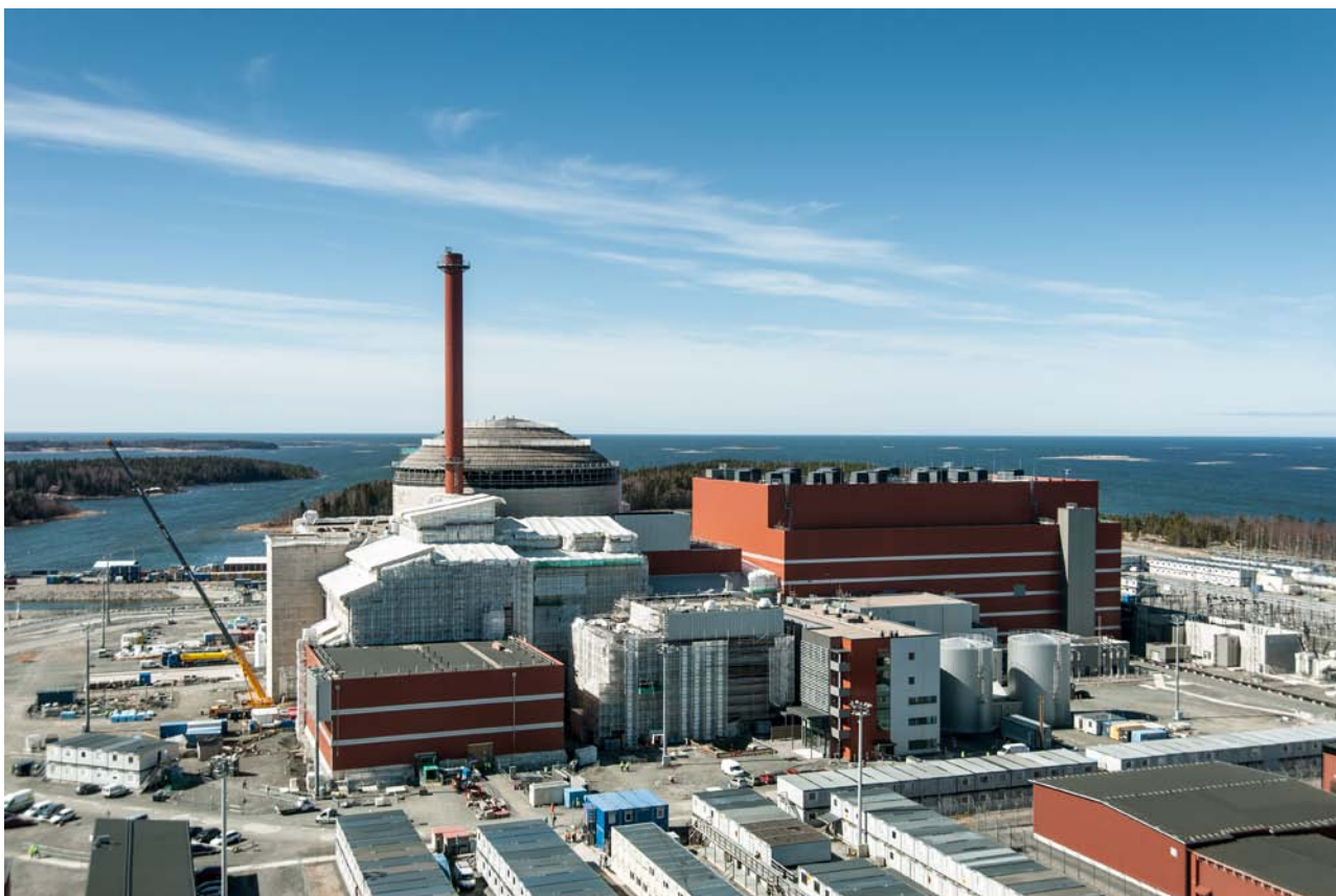
Figure 22. Olkiluoto NPP unit 3 construction site in April 2013. Source: TVO.
