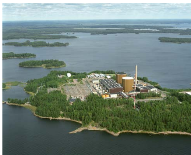
Figure 1. Loviisa nuclear power plant units 1 and 2. Source: Fortum.
