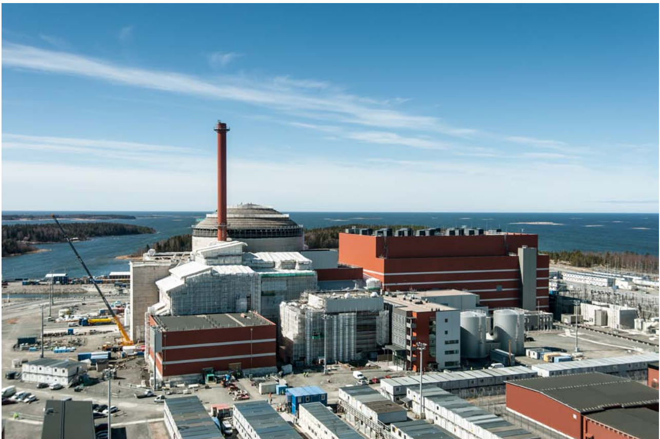
Figure 3. Olkiluoto NPP unit 3 in construction phase in April 2013. Source: TVO.
