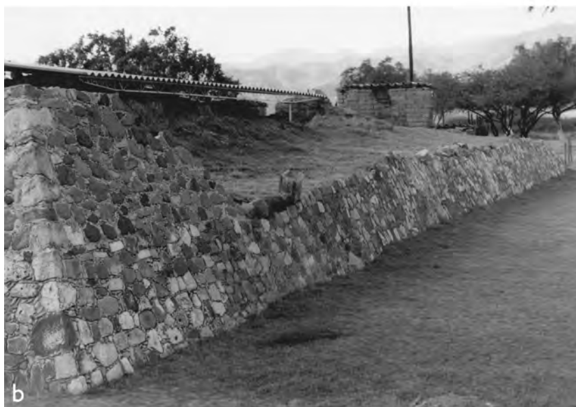
9.10. Adobe retaining walls and the east wall of Mound 195
