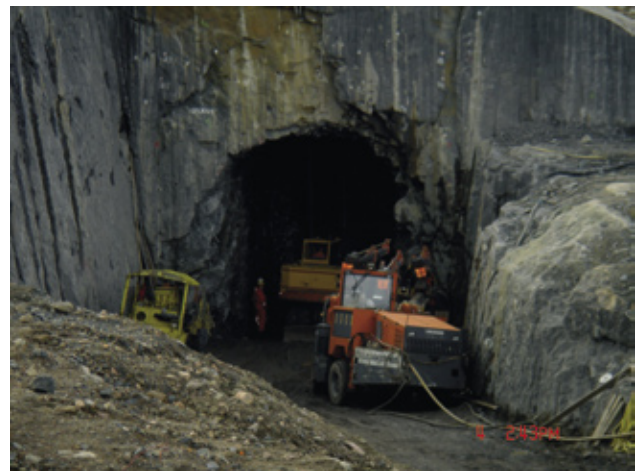
Figure 8. Underground excavation of the research galleries for final disposal of spent nuclear fuel begun in 2004.
