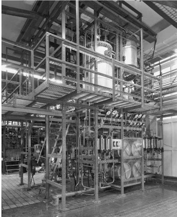
The so-called Little Hyam, an installation built in 1970 for catalysis research in relation to the HPO process. An improved catalyst was developed here.
