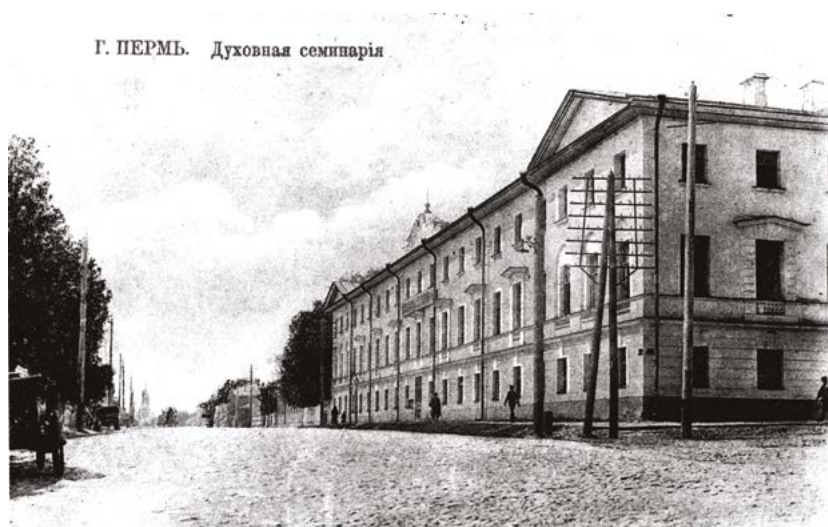
Fig. 1-1. Perm Seminary, a postcard (c.1900). This three-story brick house was constructed across a square from the city's main cathedral in 1843, after the old wooden building had been destroyed in the fire. In the mid-1930s it was completely reconstructed (with addition of two extra floors) to house an air-force school for the Red Army. Courtesy of RNB.
