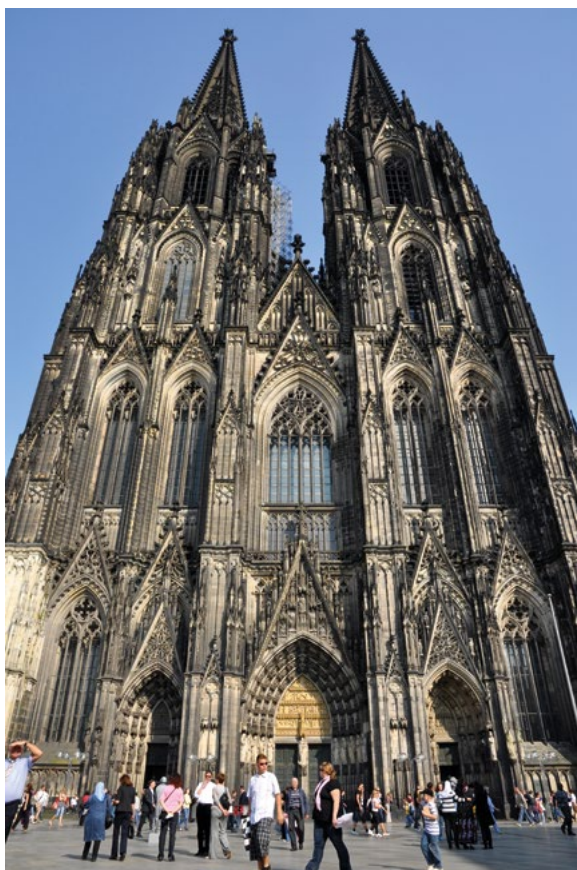
Figure 1. Example of regal architecture. Cologne Cathedral (Kölner Dom). Built 1248–1880. Photo by Tobi 87, 2009. 65
