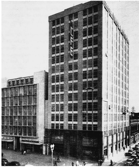
FIGURE 4.2. CFE administrative center, 1960
