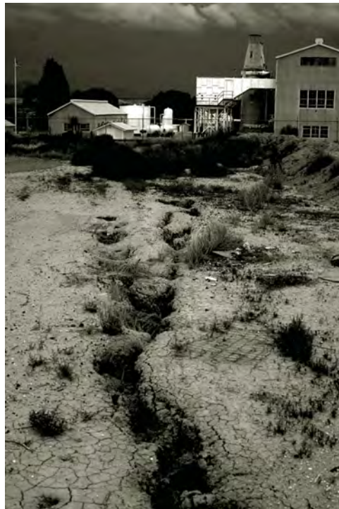
FIGURE 5.6 Subsidence crack in Benson, Arizona. (Courtesy of S.R. Anderson.)
