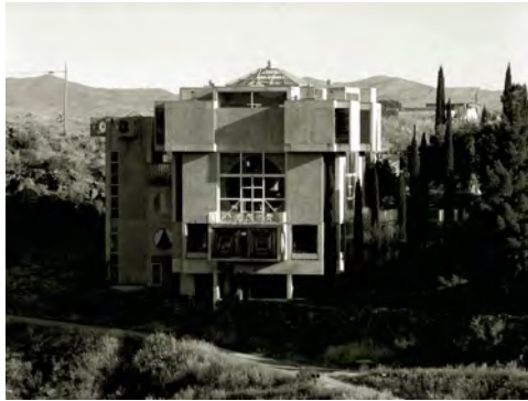
FIGURE 30.5 Crafts III building contains visitor's center, gallery, bakery, café, and residences.
