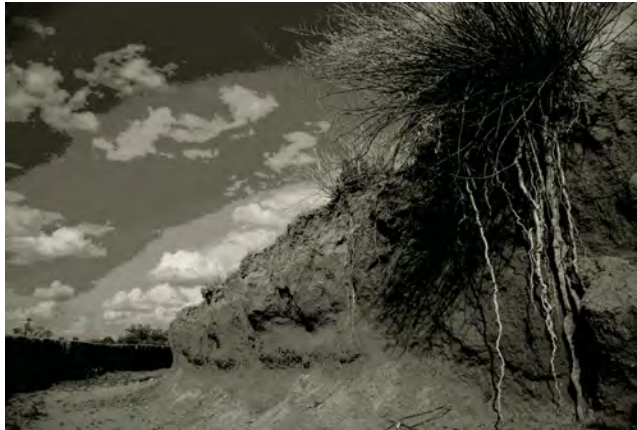
FIGURE 10.3 Degraded desert riparian wash showing accelerated streambank erosion.
