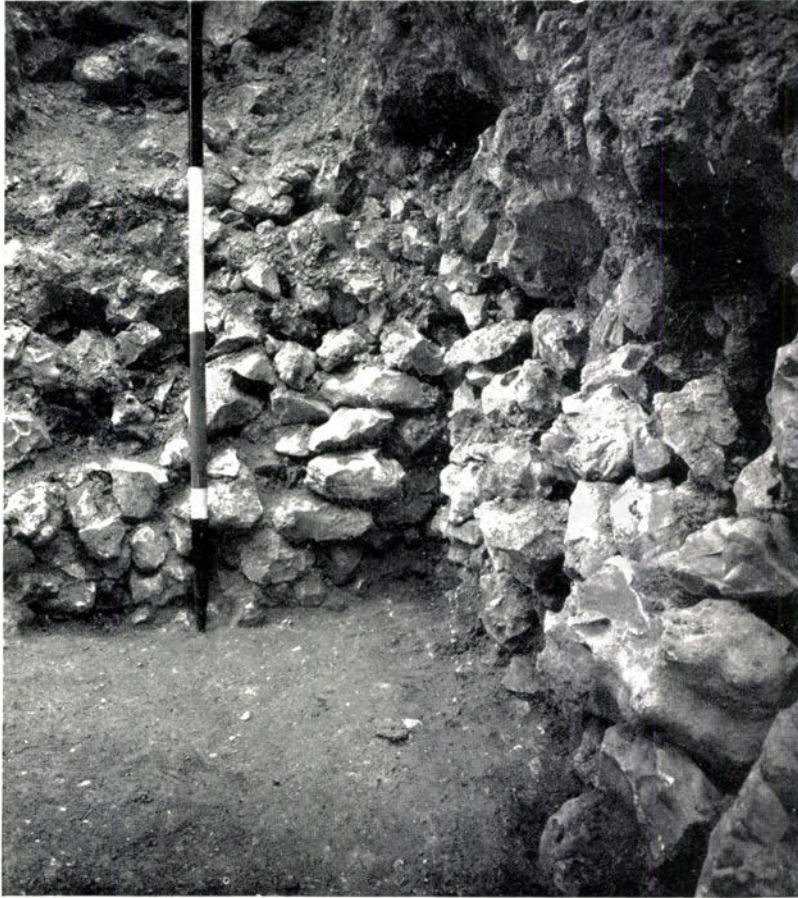
A. Flint revetment of SE. entrance (behind pole), with fallen flints across roadway in foreground
