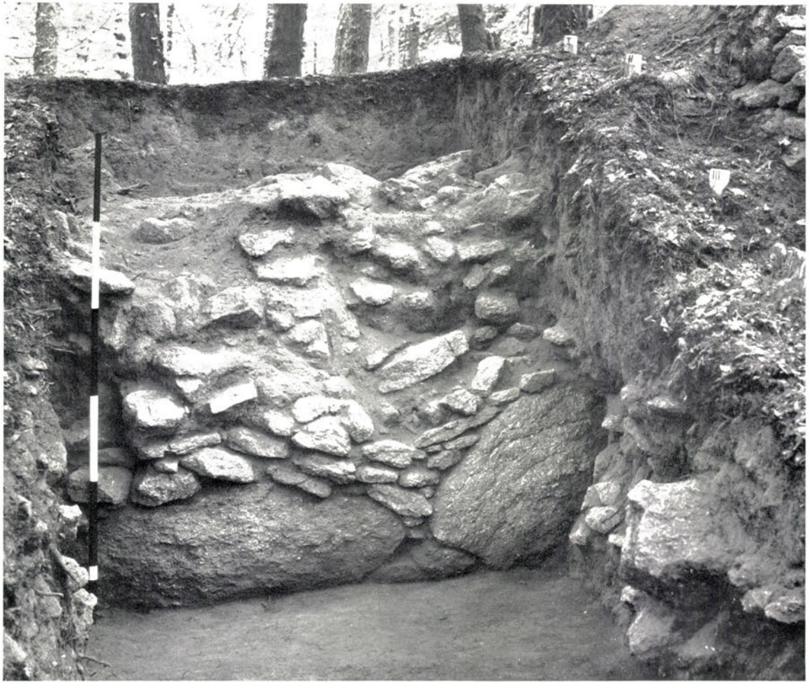
Le Camp d'Artus: Site A, showing exterior of murus Gallicus (See p. 25)
