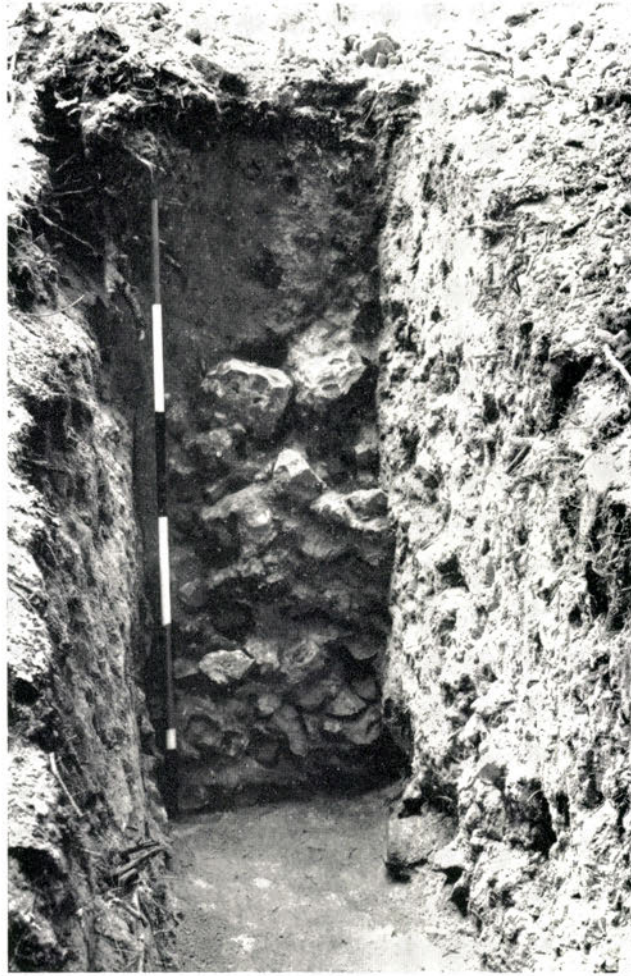
Le Camp du Canada: flint revetment of SE. entrance
