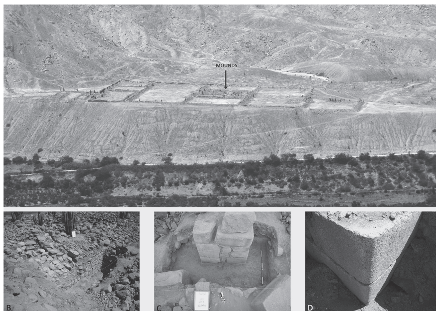
FIGURE 6.4. Photographs of Kushipampa showing (A) a northwest-to-southeast view of the ceremonial complex with indication of the location of the mounds, (B) view of the masonry of the mounds after excavations in 2008, (C) view of a megalithic doorway after excavations in 2008, and (D) detail of the finishing of the megalithic rocks used in corners of the structures. Courtesy, Hugo Ikehara.
