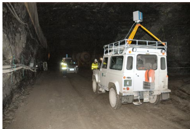
Figure 6. Laser scanning in Onkalo.
