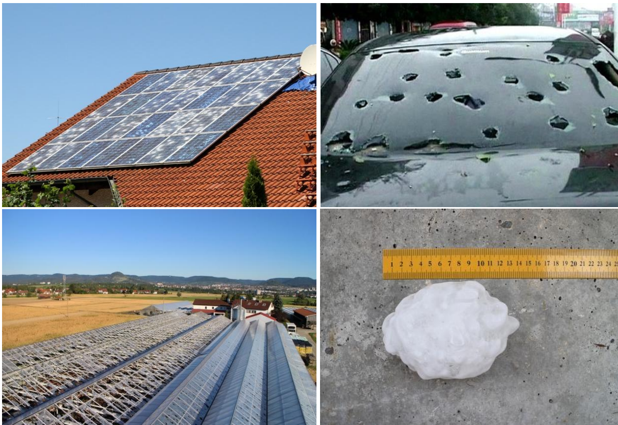
Figure 54: Images of hail damage and largest hailstone on 6 August 2013, Swabian Jura
