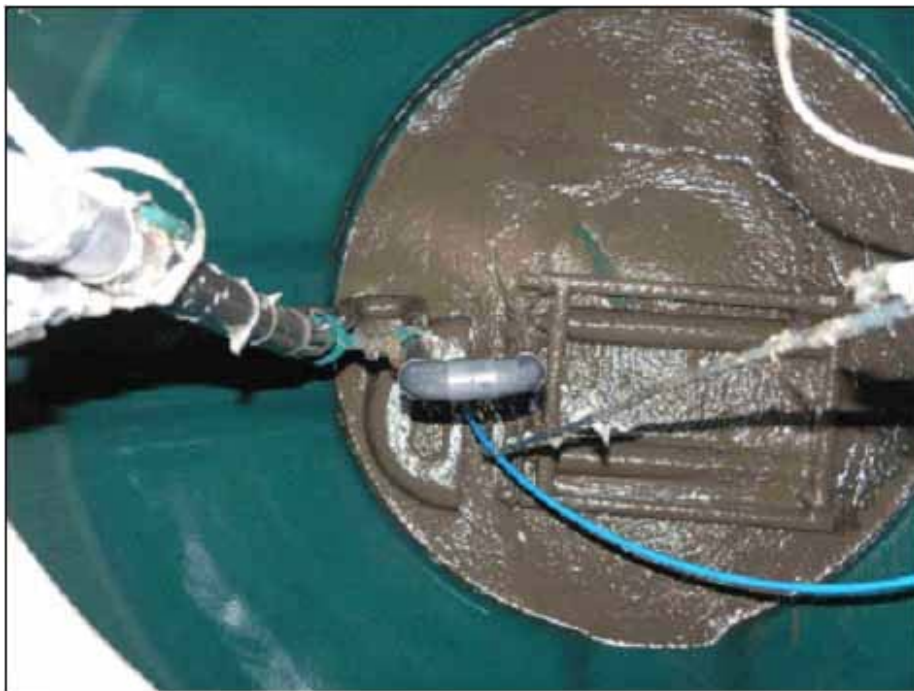
Figure 2.2 Floating scum layer inside the reactor vessel of a 'Balmoral' septic tank as viewed from above. The tubing forms part of the "air lift" pump system that transfers effluent between the chambers and pumps clarified effluent out of the system (Image courtesy of J Malley, National Trust).
