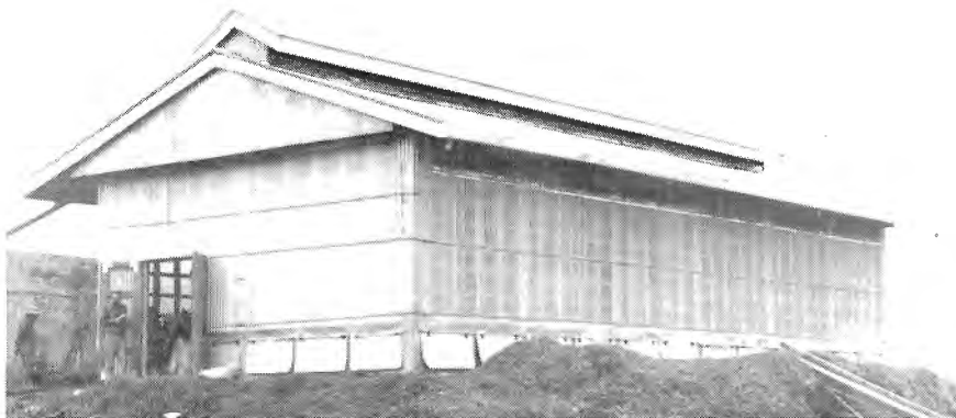
Figure VIII-2. Diffused light seed store of 100 metric tons capacity built by a group of 42 farmers in the Philippines.
