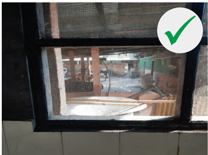
Netting in the ventilation
