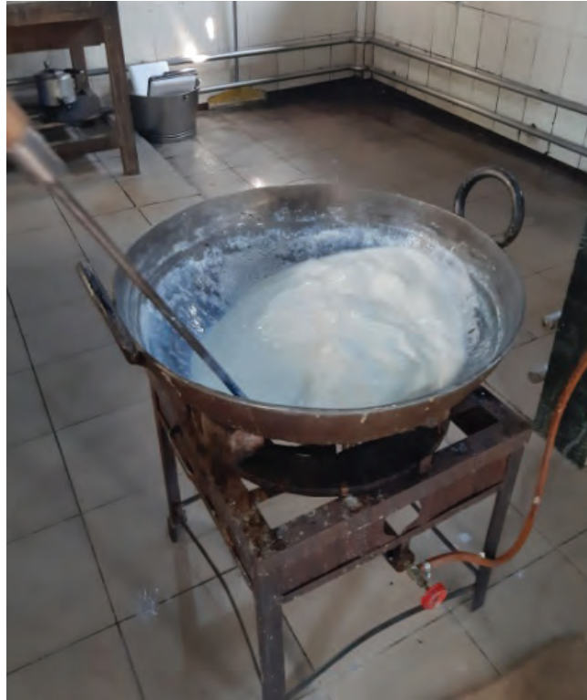
The floor is of concrete topped with good quality tiles
