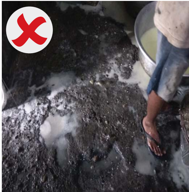
Stagnation of wastes on an uneven floor
