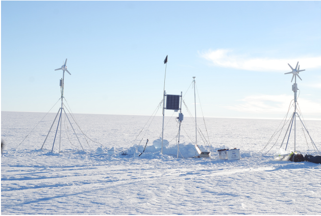
Figure 1. GNSS station installed on the Institute Ice Stream showing the two wind turbines and solar panels required to power the GNSS receiver.
