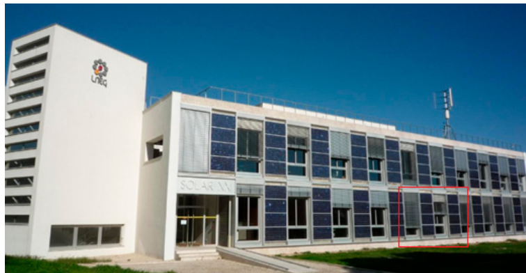
Figure 6. The Solar XXI building and the location of monitored test rooms (within the red rectangle).
