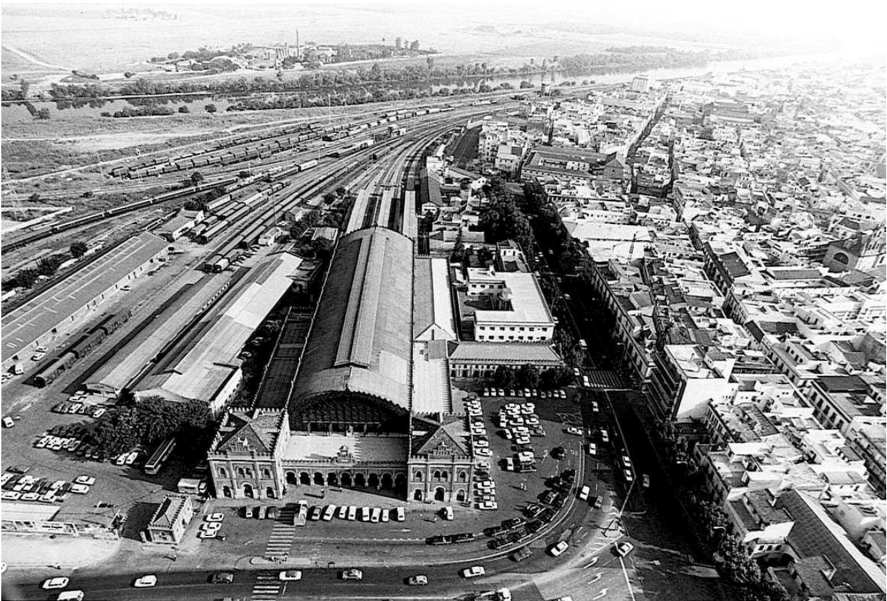
Fig. 2. Aerial view (1984) of the Plaza de Armas Railway Station (Seville, 1898-1902). The travellers' building, in the centre, is in neo-Mudejar style, on the left the workshops, the river Guadalquivir and the Cartuja-Fábrica Pickman, on the right, the historic city. Source: Diario ABC, Col. A. Esquivias, Sevilla, 2013.
