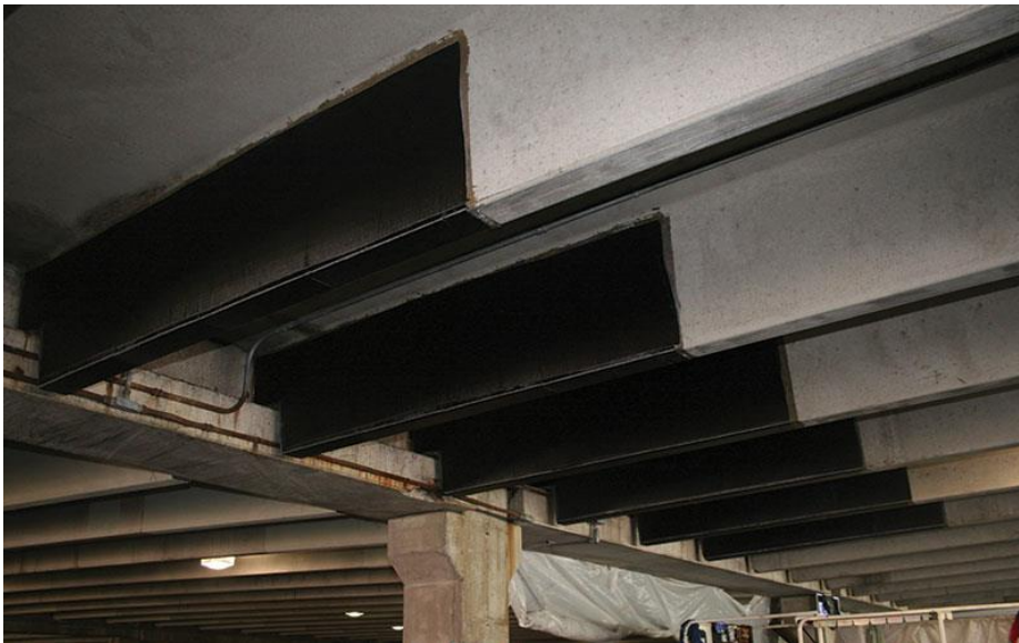
Figure 15: CFRP fabric wrapped around beams
