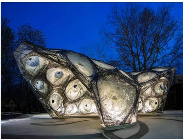
Figure 59: ITKE/ICD Research Pavilion 2013-14 made through the application of CFW [6]
