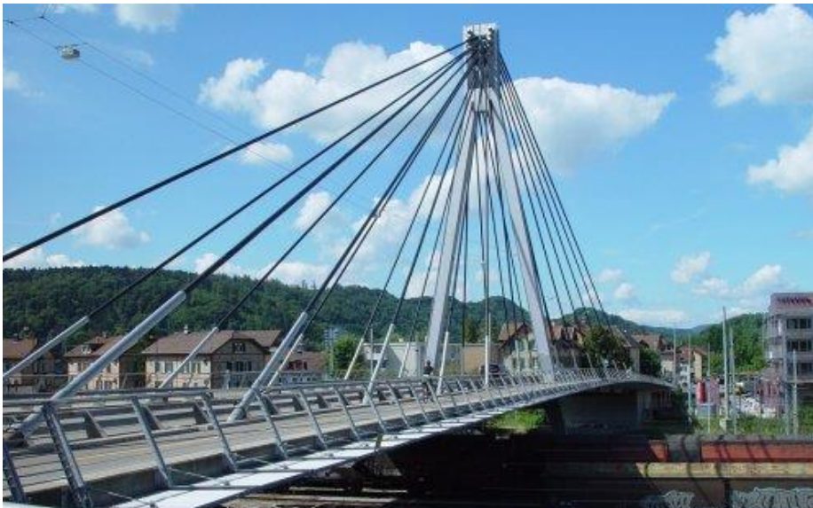
Figure 16: Stork Bridge in Switzerland, completed and opened to traffic in 1996
