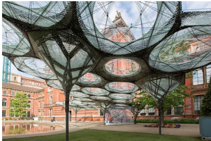
Figure 61: The Elytra Filament Pavilion also made with the application of CFW, displayed at the Victoria and Albert Museum, London, UK
