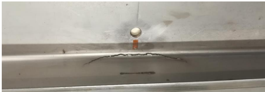
Figure 62 - Representative fatigue cracks (specimen 12 example).
