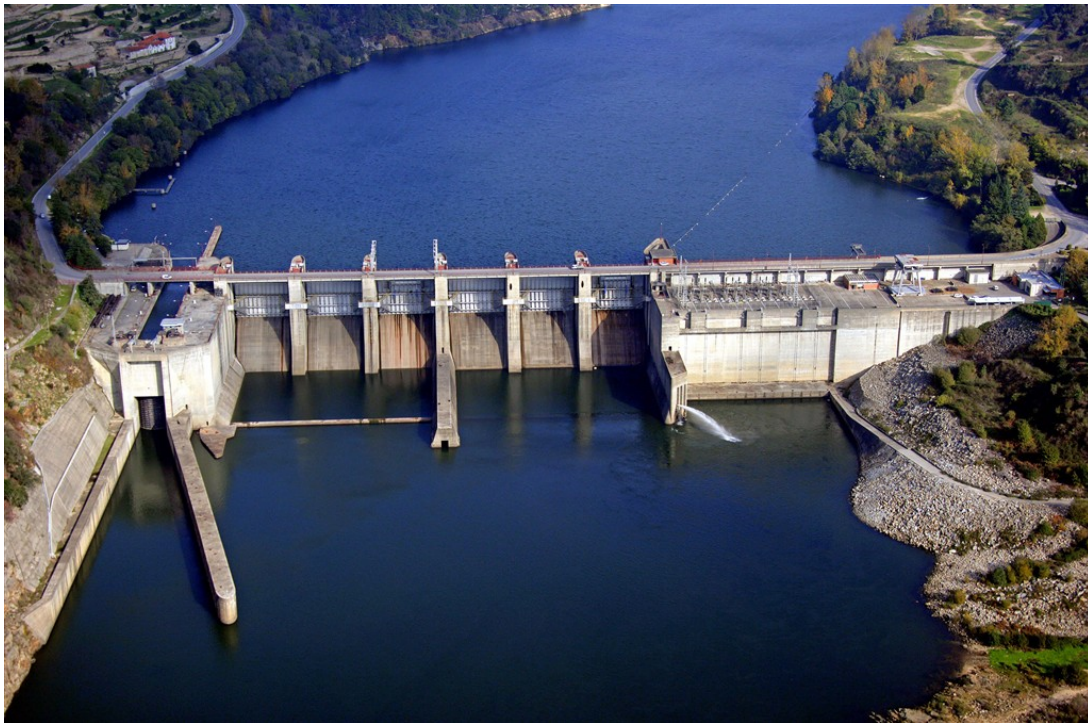
Fig. 4.22 – Aerial photograph of the Carrapatelo Lock
