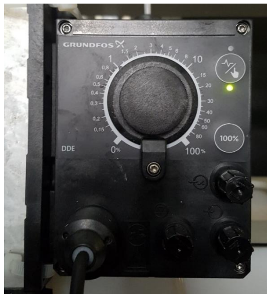
FIGURE 16 - AUTOMATIC DROPPER LOCATED AT THE BEGINNING OF THE WATER SUPPLY CHANNEL
