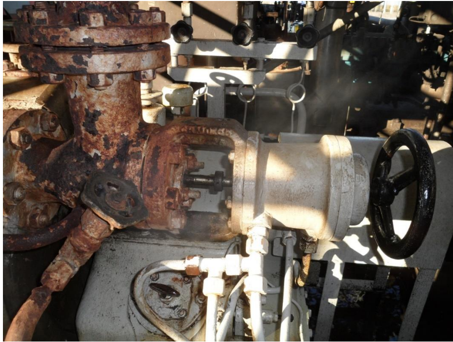
Figure 34 – Regulating Valve with Servomotor. (Hugo Araújo, 2017)
