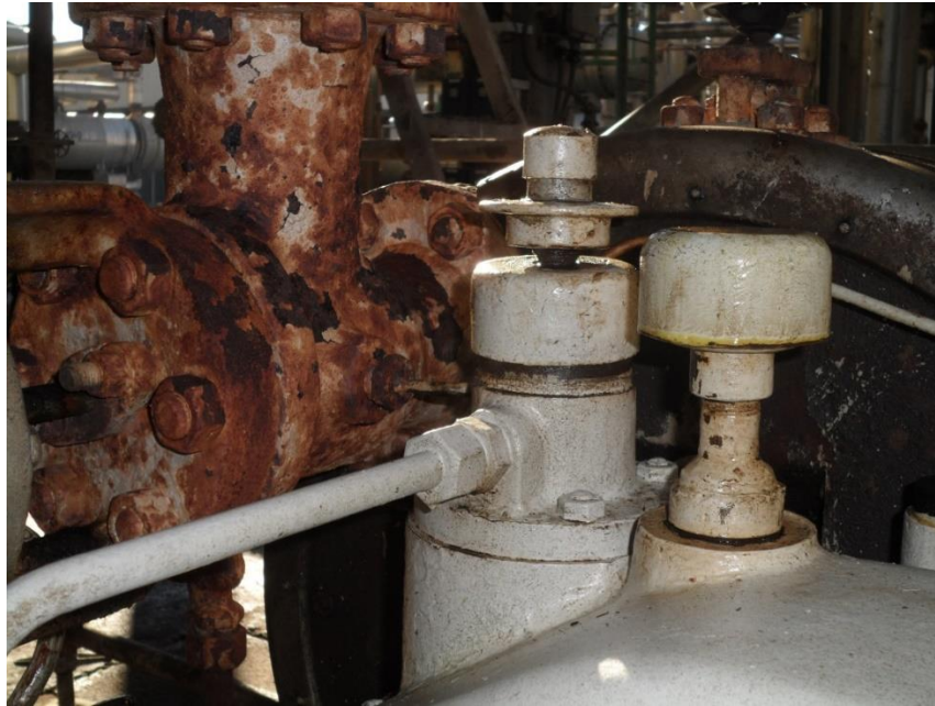
Figure 30 – Emergency Governor and Relay. (Hugo Araújo, 2017)
