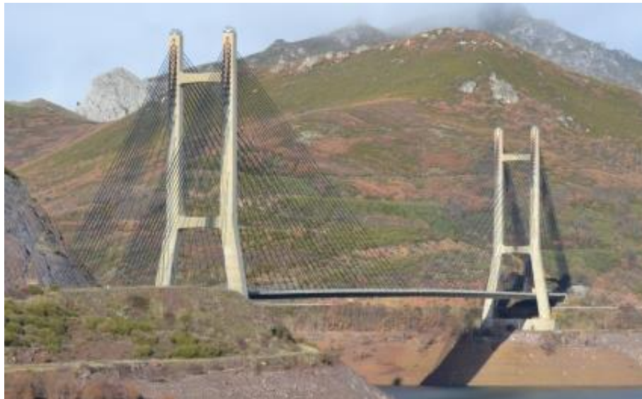
Figure 10 - Barrios de Luna Bridge (Spain, 1984)
