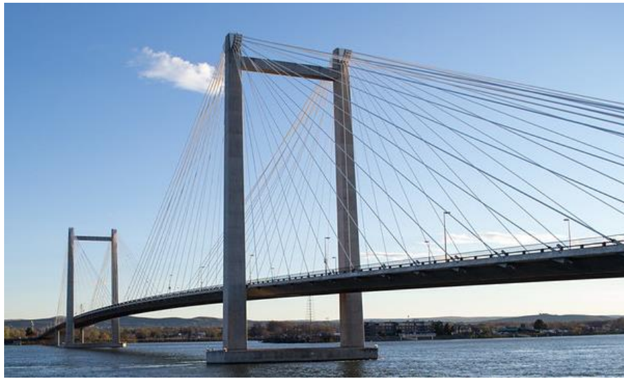
Figure 9 - Pasco-Kennewick Bridge (United States, 1978)
