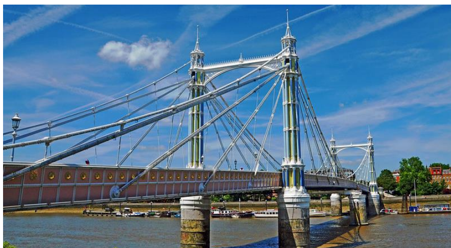
Figure 1 - Albert Bridge (London, 1873)
