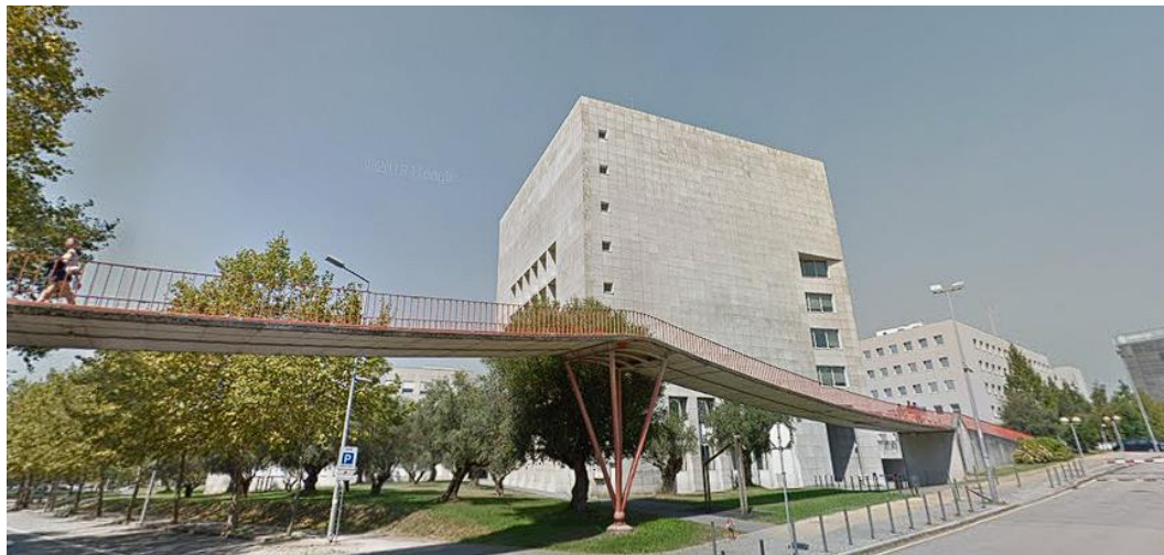
Figure 31 - Stress-ribbon footbridge at the FEUP Campus.
