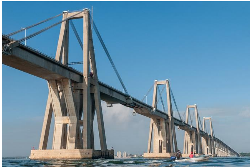
Figure 7 - Maracaibo Bridge (Venezuela, 1962)
