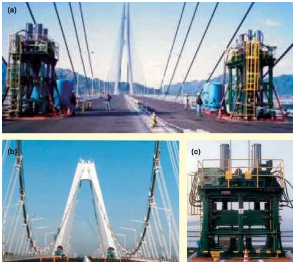
Figure 29 - Forced vibration tests: (a) Tatara cable-stayed bridge; (b) Yeongjong suspension bridge; (c) high force shaker
