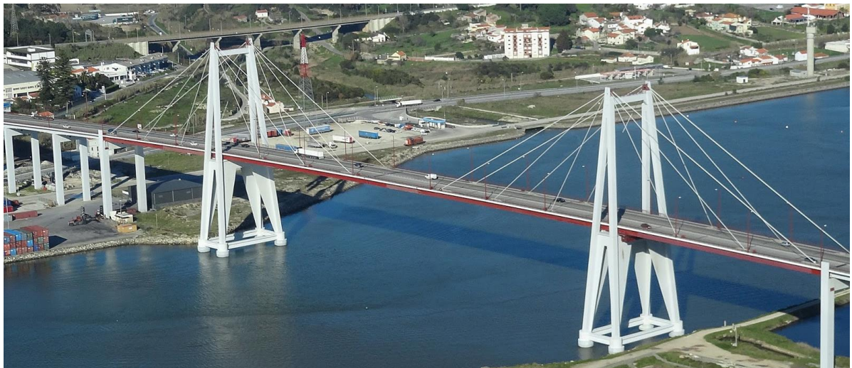
Figure 32 - Edgar Cardoso bridge, 1982.
