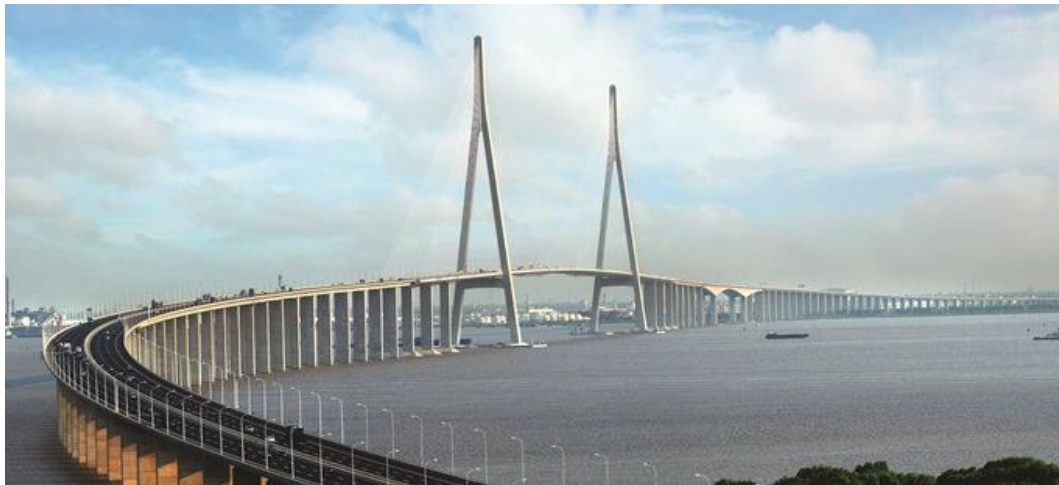
Figure 12 - Sutong Yangtze River Bridge (China, 2008)
