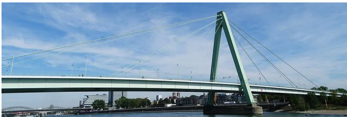
Figure 6 - Severins Bridge (Cologne, 1959)
