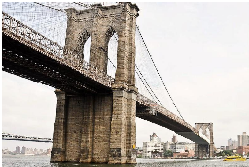
Figure 4 - Brooklyn Bridge (New York, 1883)
