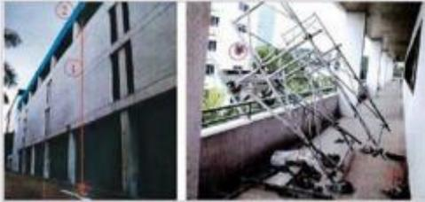
(1) Falling Accident Direction, (2) Roof Painting Area, (3) The Castor Wheels, (4) The Scaffold with Cantilever
