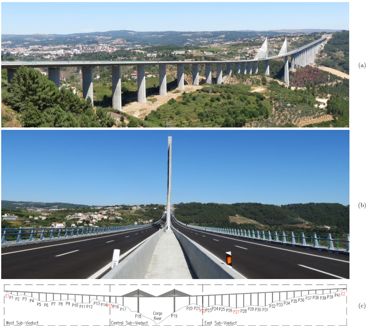
Figure 3.1 – Corgo Bridge: (a) general view, (b) general perspective of the deck and (c) side elevation.
