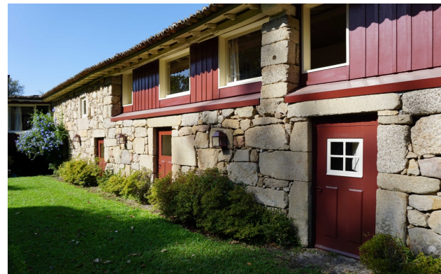
Figure 4. Façade facing the backyard.
