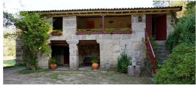
Figure 3. View of the west façade.
