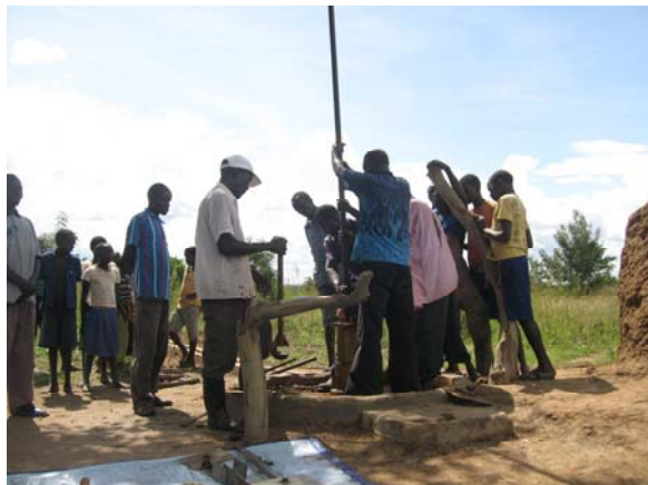
Dis-assembly of a water point in Katakwi District; the fieldwork relied on strong support from and engagement with the local communities
