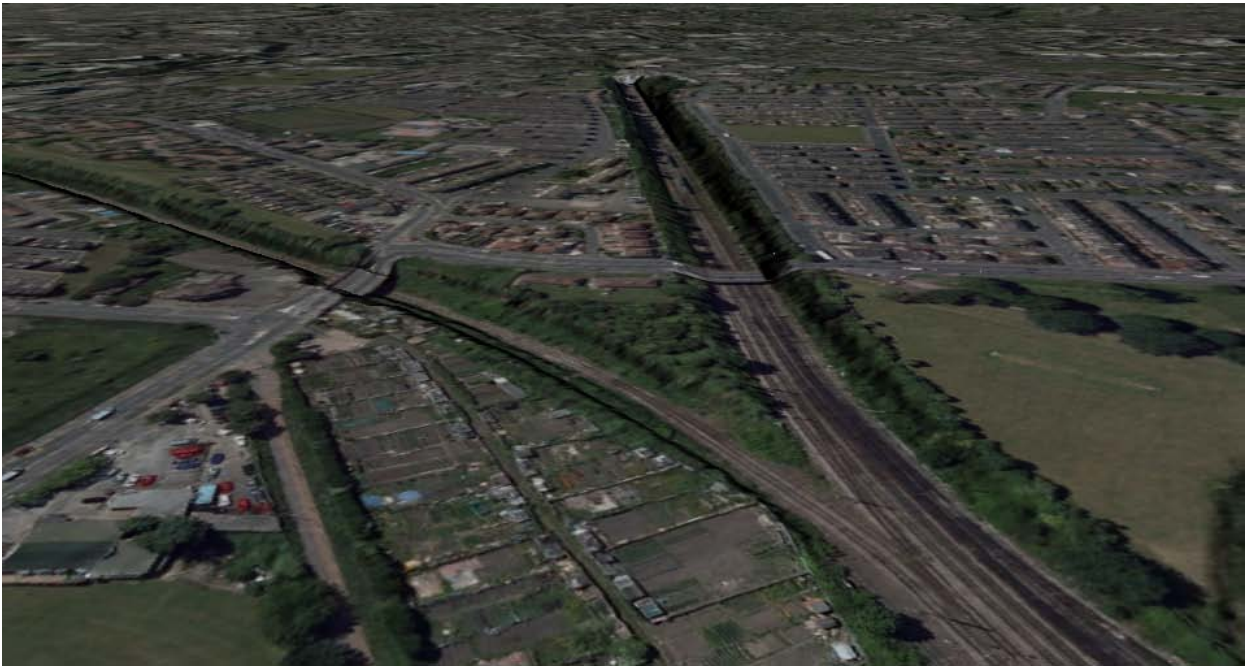
Figure 11 LiDAR with Aerial photography revealing the rail cutting
