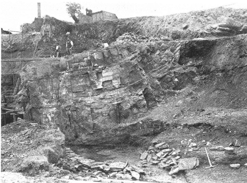
Plate 6 Ganister quarry in Stanningley Rock, showing beds folded up against a fault, near Meanwood Road in 1894. (British Association for the Advancement of Science Photographic Collection.)
