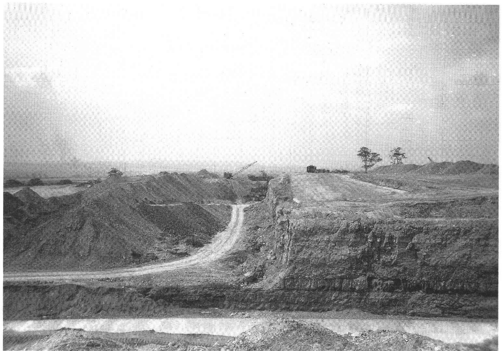
Plate 10 Spring Wood opencast coal site [348 318] as seen in 1945: backfill area to the left; excavation in the Middleton Little Coal far centre.
