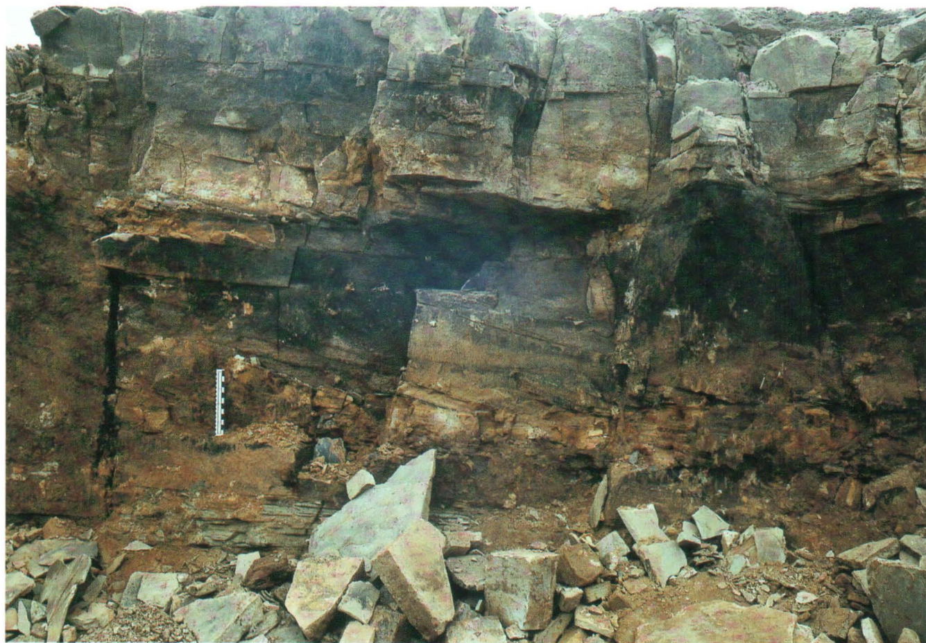
Plate 1 Rough Rock Flags exposed at Woodside Quarry [2564 3853].
