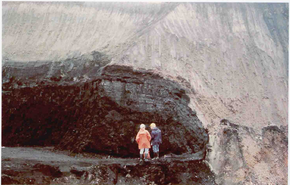
Plate 3 Exposed face of the Thick Coal at the Dibdale Road opencast coal site. Note the collapse of overburden, including redened, burnt shale into old workings on the right.
