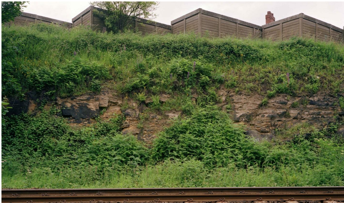
Figure 4. Railway cutting (north side) at Killingbeck, Leeds [NGR 434680 434150] in the Slack Bank Rock, Pennine Lower Coal Measures Formation. The sandstone comprises ~6m of fine-grained sandstone which tends to be massive in lower parts and cross-bedded above. Photograph taken in 1991. BGS GeoScenic archive no. P213856.
