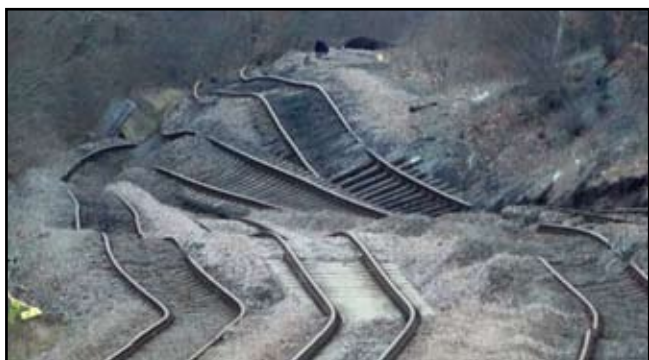
Figure 5. The landslide failure, mainly of colliery waste, impacting the railway from Doncaster at Hatfield Colliery in February 2013 (photo: BGS, NERC).
