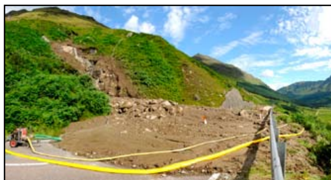
Figure 2. The debris flow that dumped superficial colluvium onto the road over the Rest and Be Thankful Pass in Scotland in October 2013 (photo: BGS, NERC).
