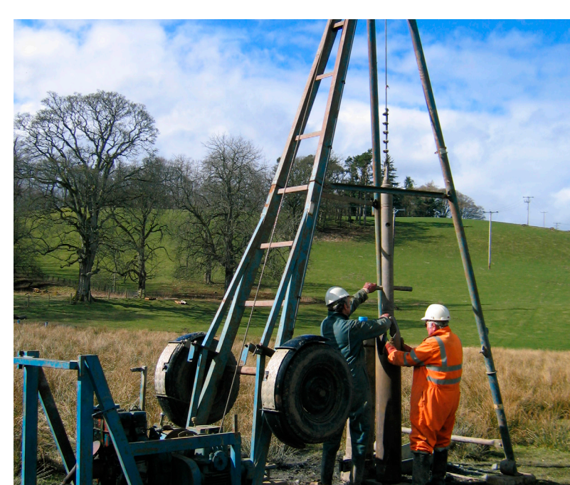
Drilling to install groundwater boreholes.
