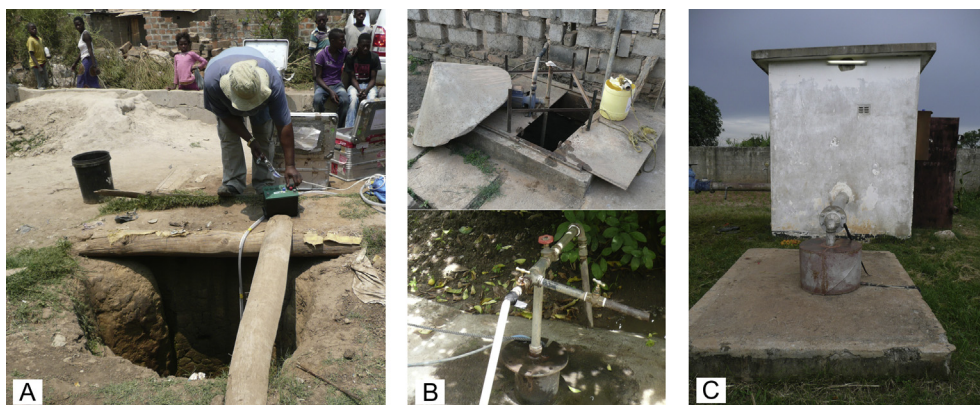
Fig. 4 – Relating groundwater source vulnerability to land use (a) vulnerable unlined shallow well (K34) adjacent to the road in lower cost housing area, (b) shallow well (K20) and borehole (K18) with protective headworks located in gated properties within higher cost housing areas (c) fully sealed public water supply borehole within secure compound in the peri-urban Mukobeko wellfield.
