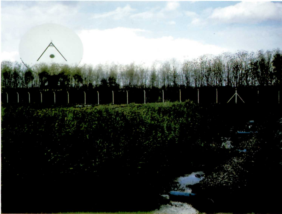
Plate 17. New technology sewage treatment? A reed bed treatment system at Kingstone and Madley (Welsh Water Authority)
