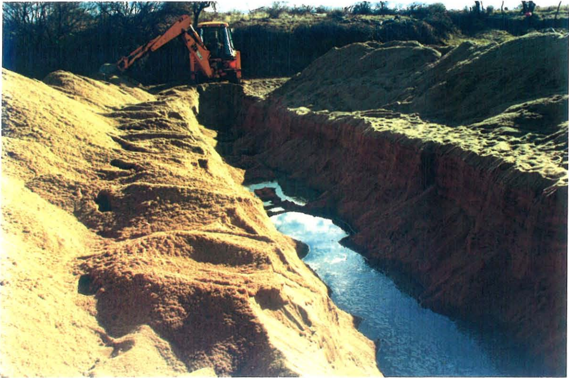
Figure 34. Excavation of geological inspection trench to water table at Gulubane.
