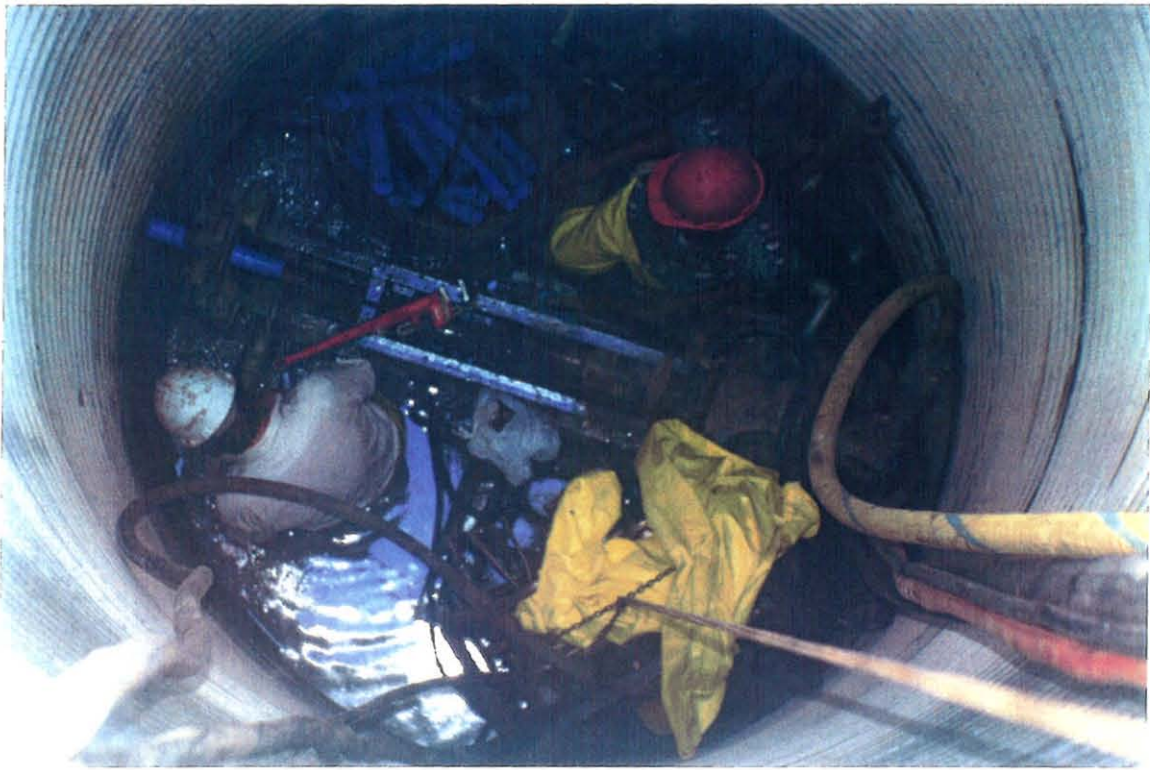
Figure 22. Installation of 2" screens and pipes.
