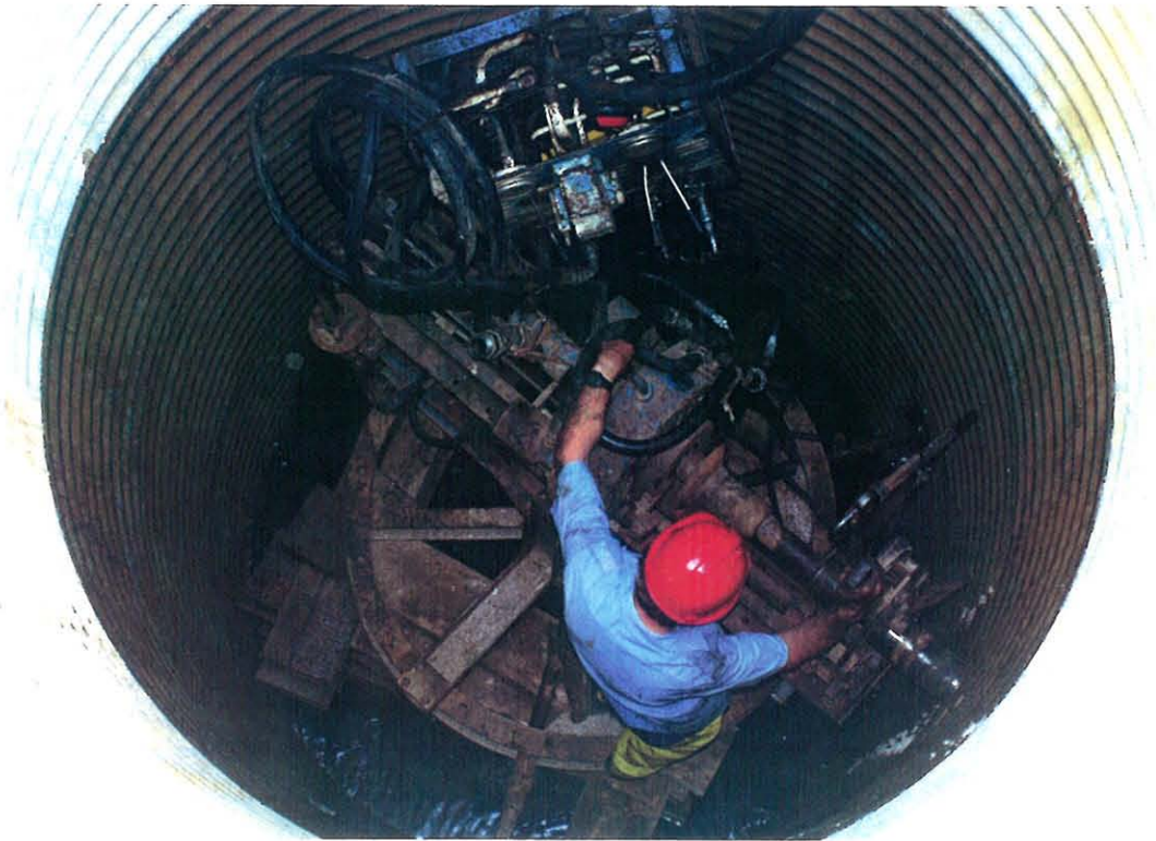
Figure 20. Initial drilling through the well-shaft casing using a U100 core bit faced with tungsten carbide clusterite chips. Note rig positioned upon a stack of timbers
