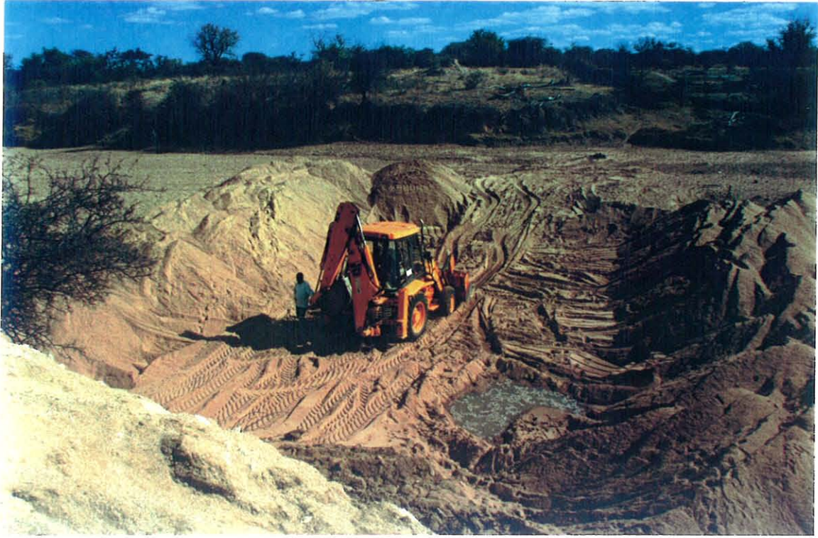
Figure 31. Excavation of main dewatering trench to water table at Gulubane.
