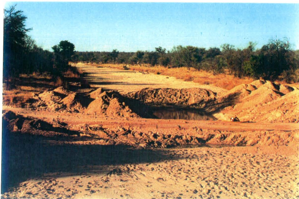
Figure 2. Water abstraction for rural road construction from a mechanically dug hole in the bed of the Ntshe sand-river
