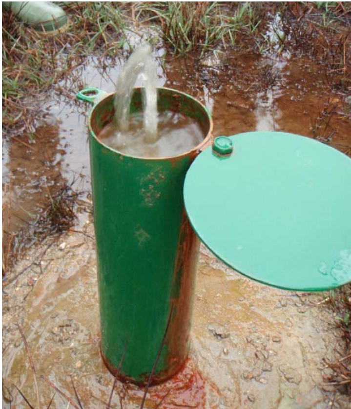
Figure 2. Piezometer 'BD2' showing artesian groundwater pressure (12 th January 2011)
