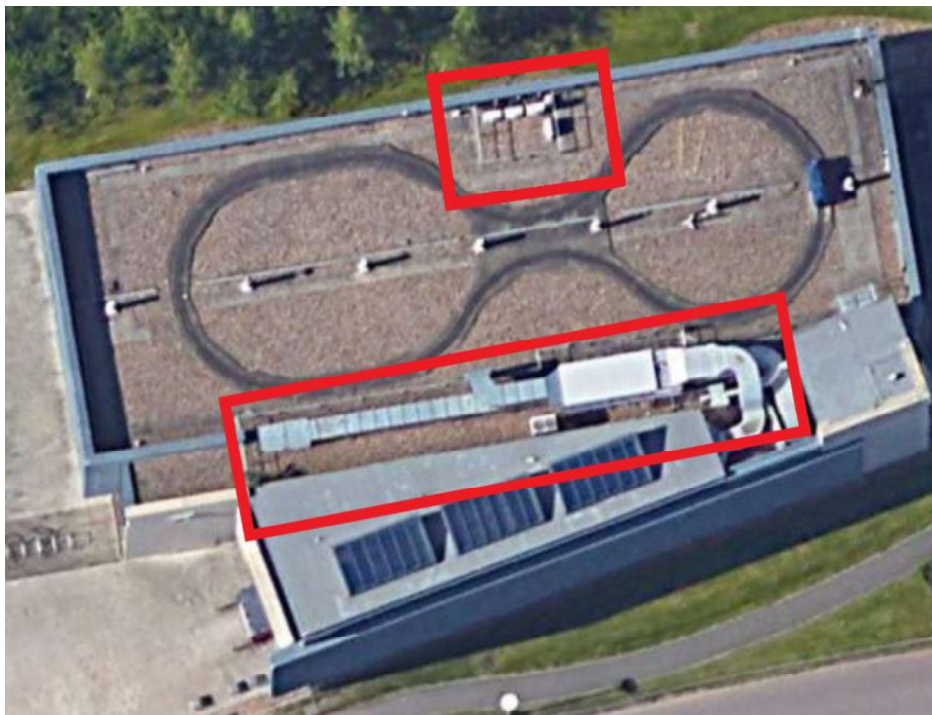
Figure 5.6 Nottingham Geospatial Institute Trial Site Top View
