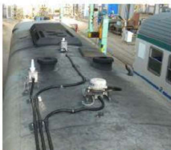
Figure 2 Antennas placed in ALN 668 3114 roof (Courtesy of ASTS)
