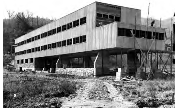
7-8 Construcción del Studies Building proyectado por Lawrence Kocher y materializado en hormigón armado, piedra local y revestido con chapa de acero galvanizado, 1940-41. / Studies Building construction designed by Lawrence Kocher and materialized in precast concrete, local stones, and coated with galvanized steel. Fuente / Source: Western Regional Archives, State Archives of North Carolina (WRA/SANC).
