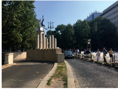
2. The spatial position of the memorial, squeezed in between roads, author's photo, July, 2014
