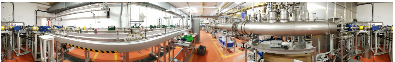
Figure 8.1.: Cylindrical panorama composite of the S-DALINAC main accelerator hall. On the right side one can see the helium vessels of the super-conducting main linear accelerator. On the left side three recirculation beamlines are visible. Dipole magnets are painted blue, quadrupole magnets are yellow and green. (Picture taken in April 2019)
