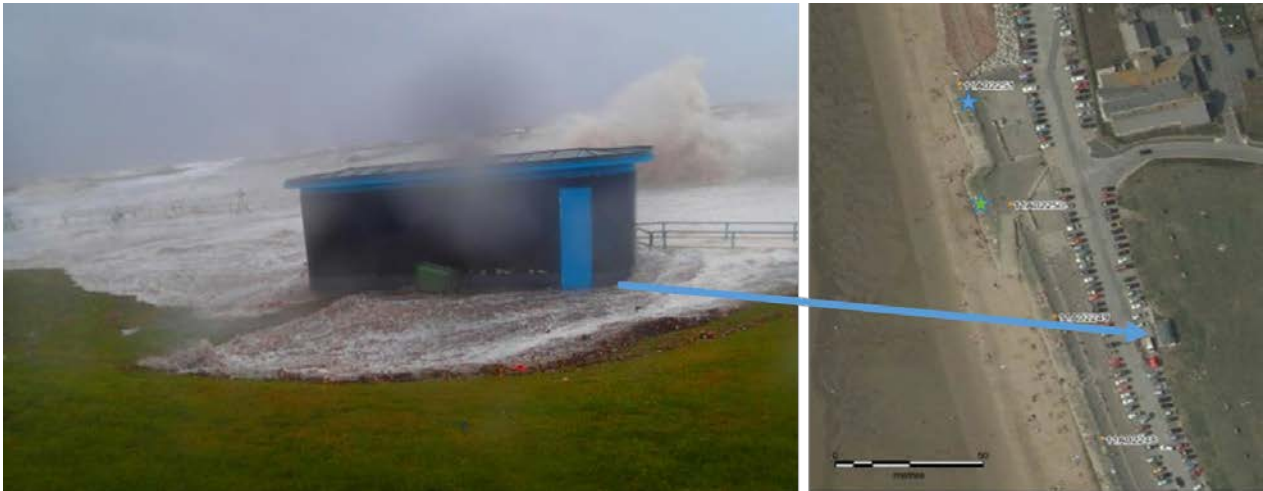
Figure 2.1: The Crosby sea wall frontage, 5 December 2013 (left) and the northern section of the car park at Hall Road (right). Images provided by the Sefton Council. The blue star marks the WireWall deployment location on the promenade and the green star the start of the survey line where numerical estimates were generated on the slipway. The slipway has a similar cross-shore profile to the promenade but is advanced slightly seaward of the main defence line.
