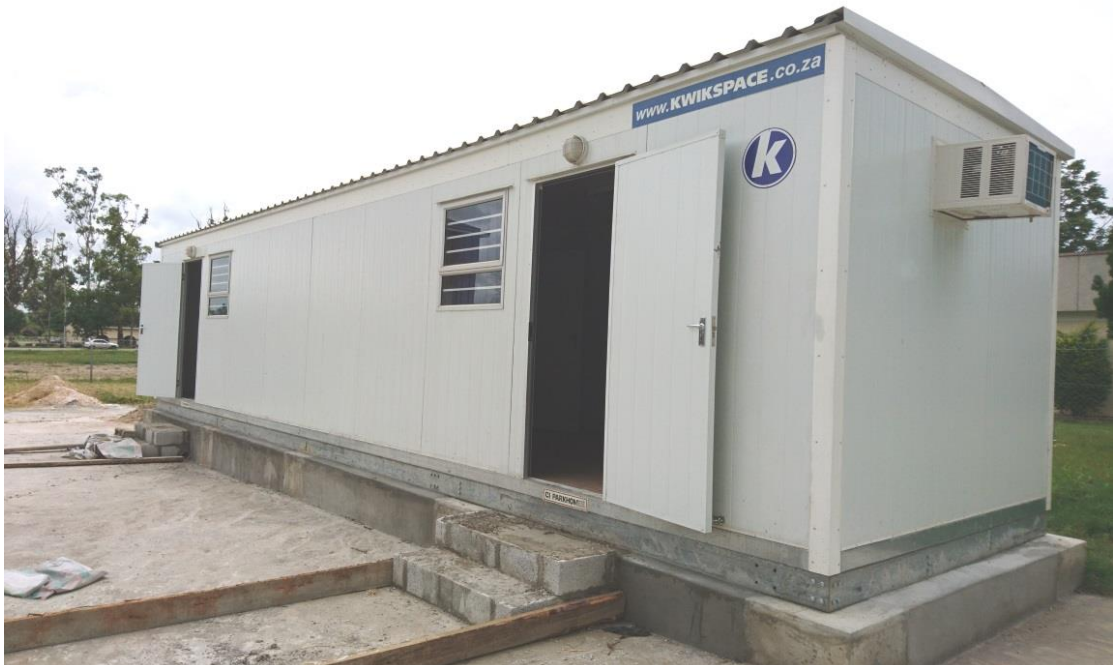
Figure 7: Solar energy centre of excellence construction site, January 2018
