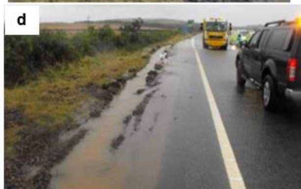
Figure 6 | (a) deposition of eroded soil particles from surrounding farmland migrating into HFDs, (b) RDS, rich in large particles, migrating towards the edge of the road (c) completely clogged HFDs running parallel with CCRSB, (d) ponding on trunk roads and HFDs.
