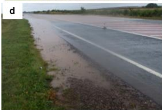
Figure 6 | (a) deposition of eroded soil particles from surrounding farmland migrating into HFDs, (b) RDS, rich in large particles, migrating towards the edge of the road (c) completely clogged HFDs running parallel with CCRSB, (d) ponding on trunk roads and HFDs.
