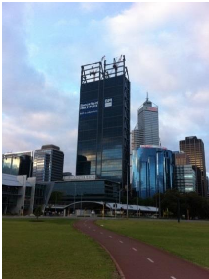
(a) Completed building
