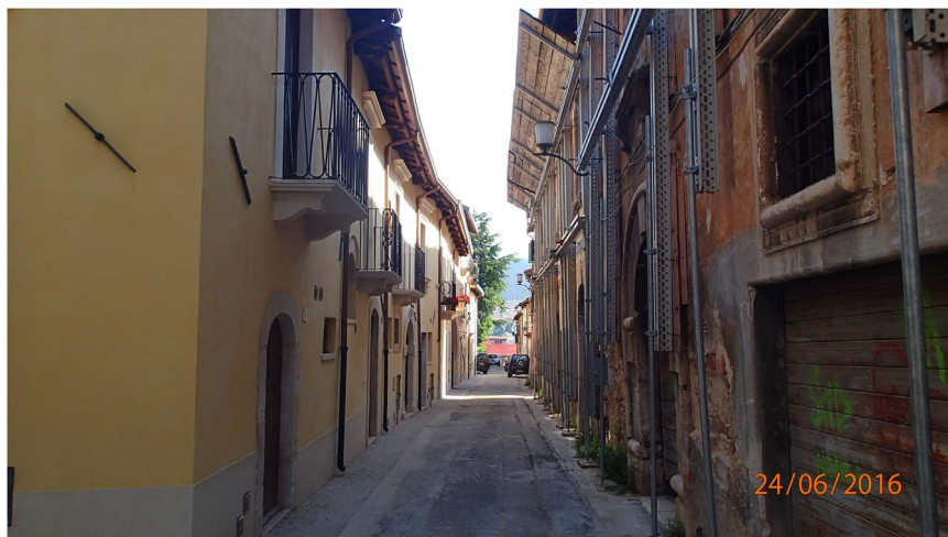
Fig. 11. Contrasts in the recovery process of the city center in L'Aquila.
